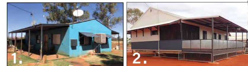
1. Block wall house with a slab on ground (Heavy-weight house) 2. Framed house built off the ground (Light-weight house)
